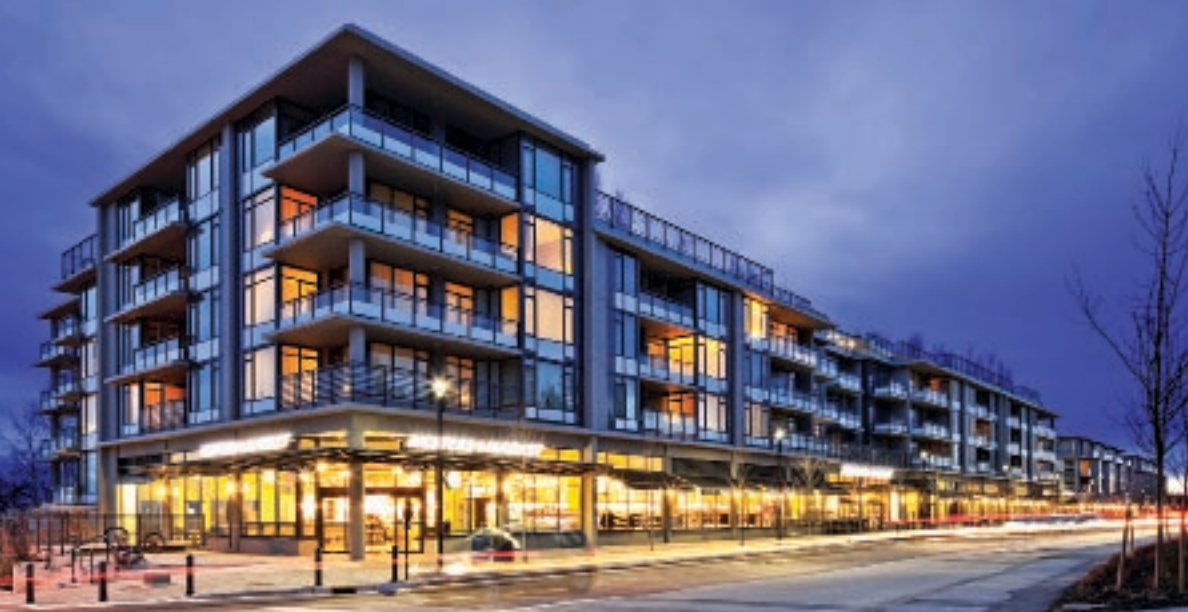
The Hub at Simon Fraser University is LEED-certified, uses geothermal heating and cooling, and incorporates green roofs at various levels. Photo by Derek Lepper, courtesy Neale Staniszki Doll Adams Architects.
