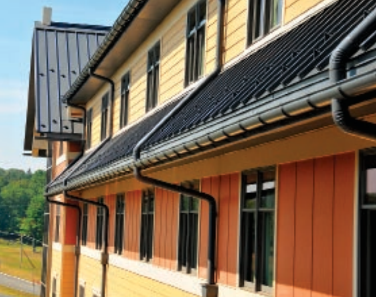
Firestone 24 gauge UC-3 Una-Clad™ metal panels in Charcoal Gray installed on the Mount Airy Casino and Hotel, Mount Pocono, Pennsylvania.
