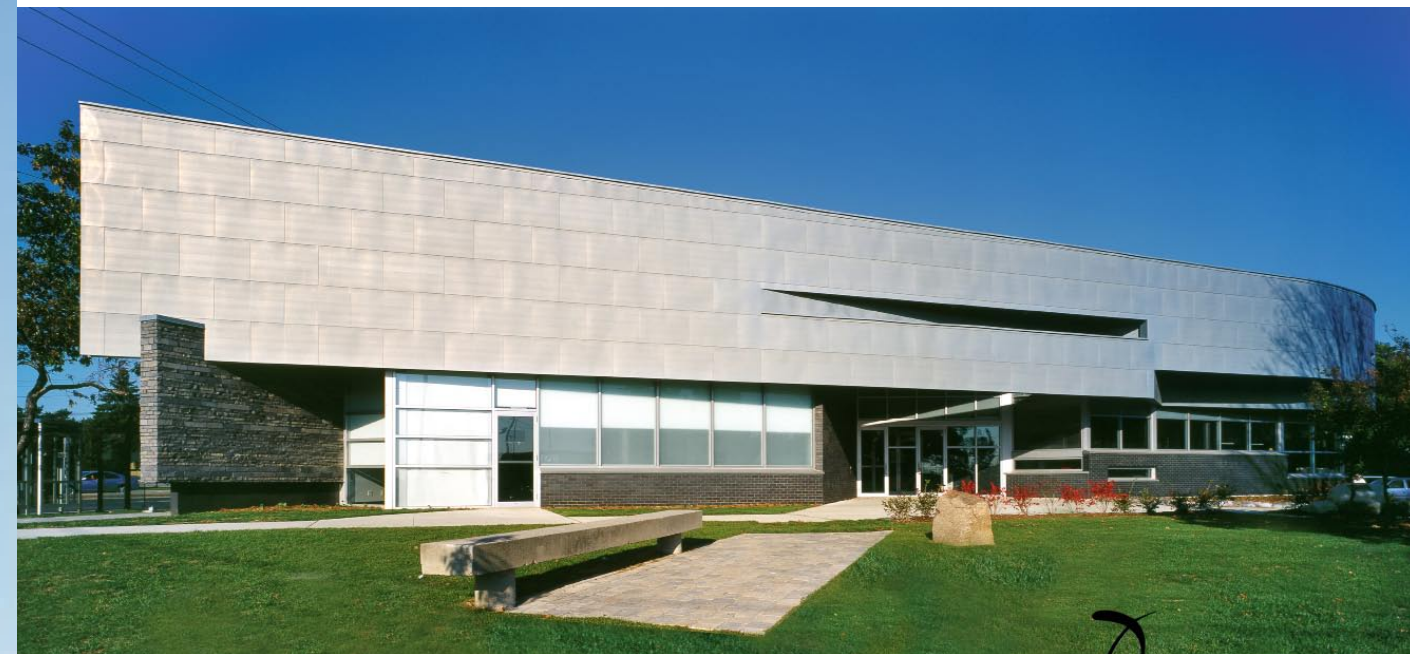
PHOTO COURTESY OF ENGINEERED ASSEMBLIES INC.
