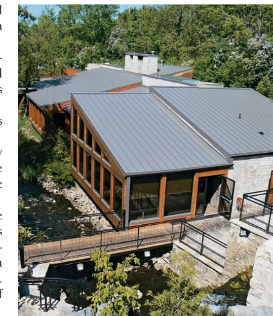
PHOTO COURTESY OF JOHN KENYON LIMITED AND VICWEST
